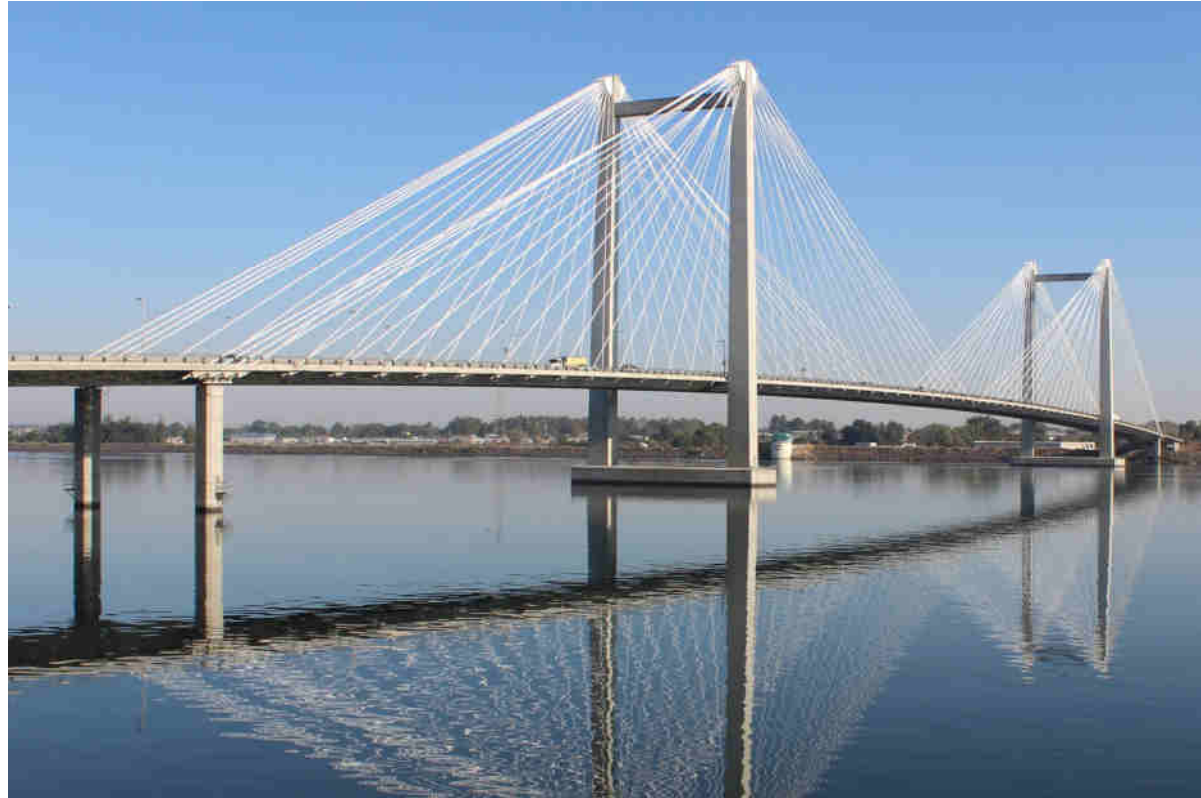
Ponte Pasco Kennewick
