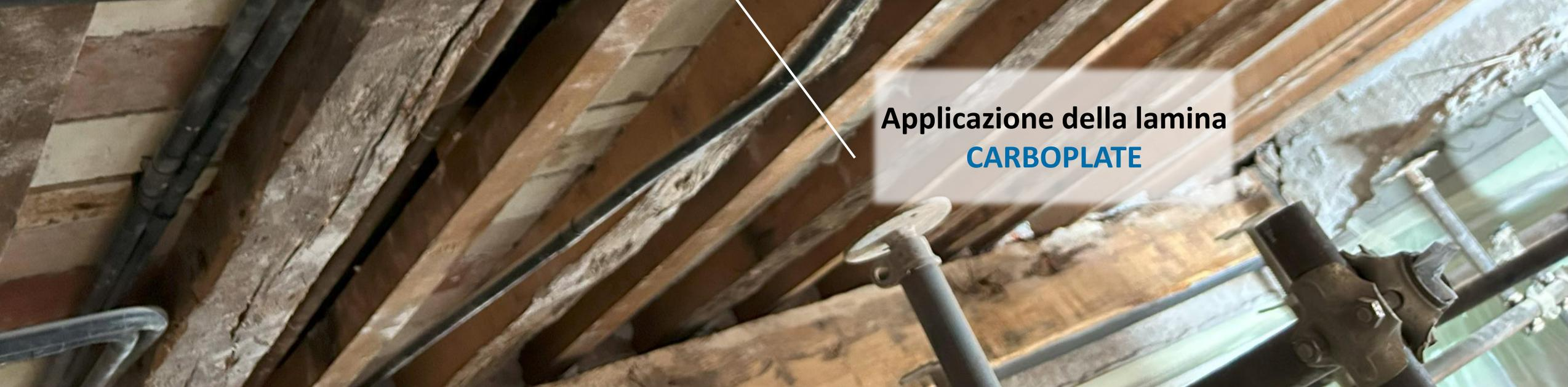
A photograph showing a dark grey carbon plate being applied to a wooden structure. A white line points from the text box to the carbon plate.
