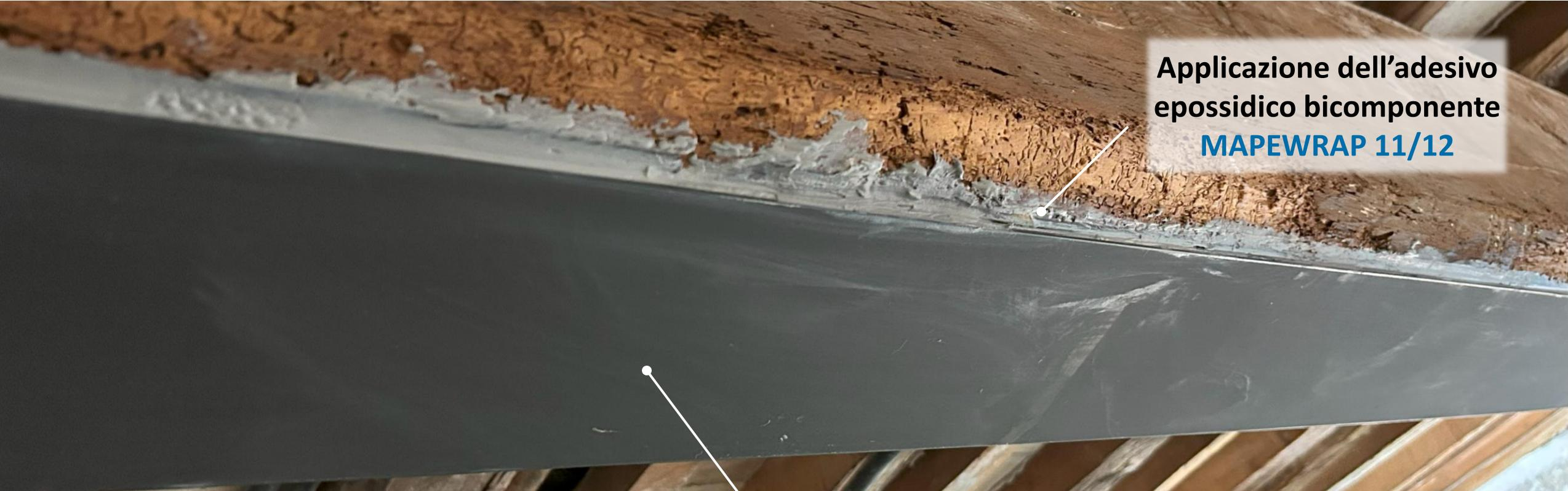
A close-up photograph showing a grey adhesive being applied to a rough, brown wooden surface. A white line points from the text box to the adhesive application.
